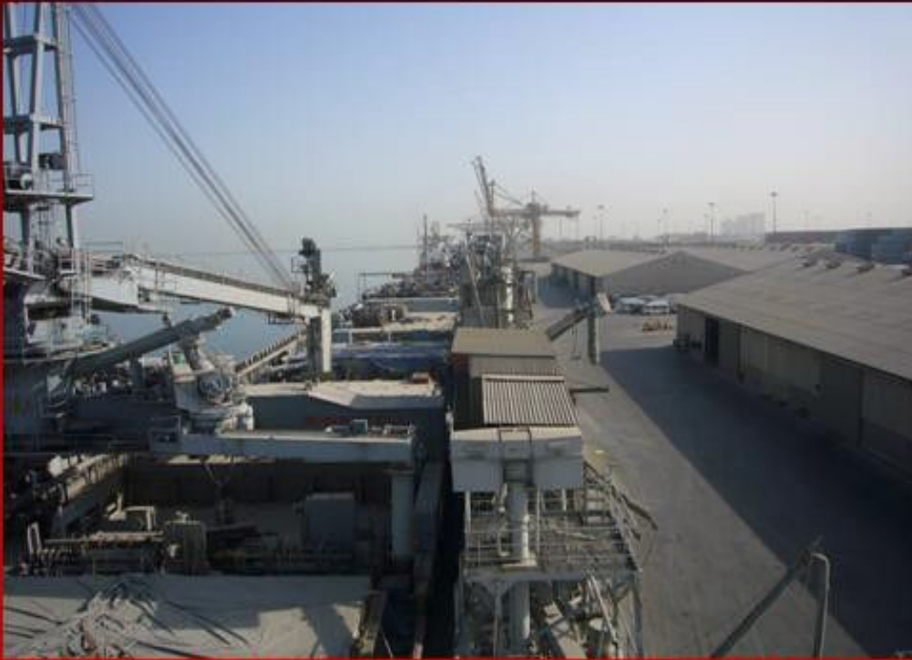
Floating Silo – Berth Side
